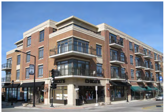
New Construction, Mid-Scale Storefront Building
