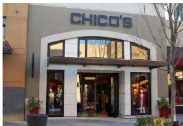
Commercial Grade Doors & Windows on Commercial Buildings.
