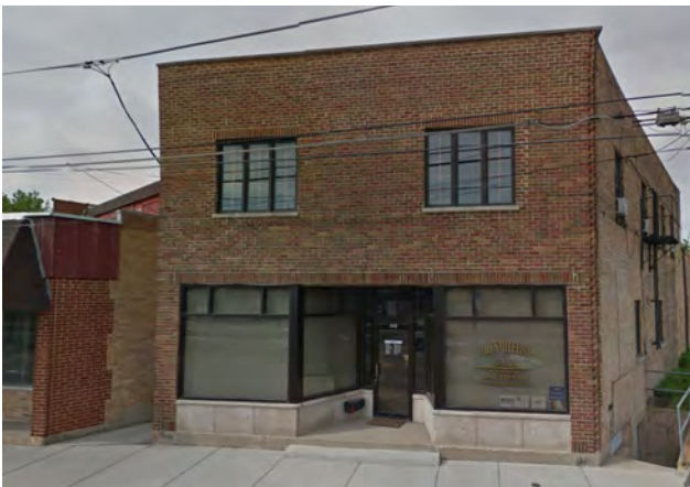
Existing Historic Storefront Building
