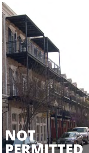
Balconies: Covers More than 40 Percent of Facade
