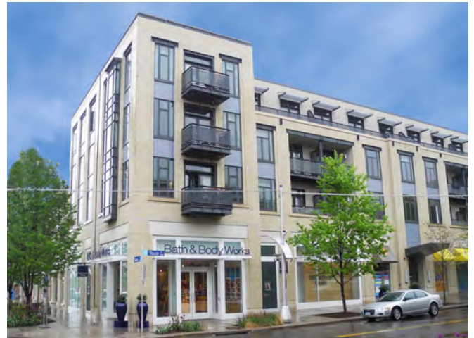
New Construction, Mid-Scale Storefront Building
